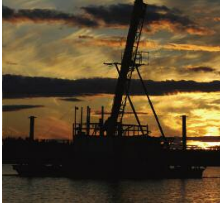
Barge with Drill Rig
